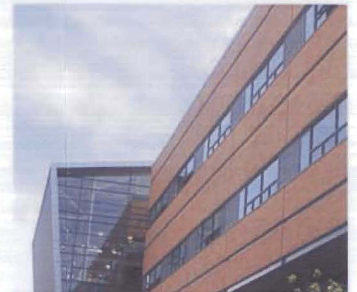
Brick Facade with Ribbon Windows
