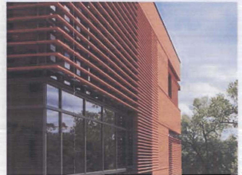
Sunshading and Curtainwall
